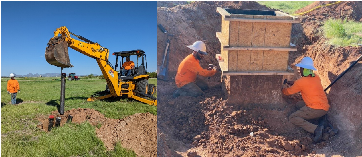
Excavating the soil cores and monolith from the Davis Monthan AFB (Tucson, AZ)
